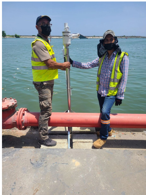
Storm surge gauge installation in Dominican Republic.
